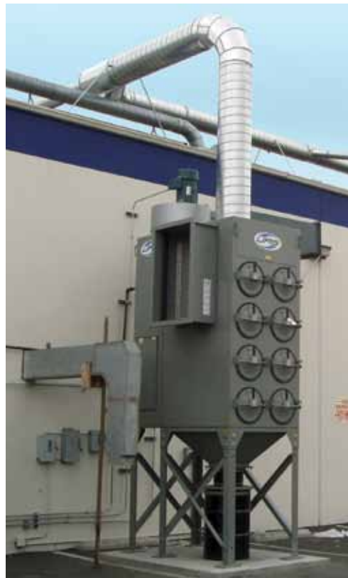
SFC 16-4 used for blending nutritional powders.
